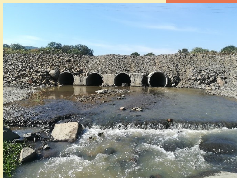
Existing Pipe Culverts on P280
