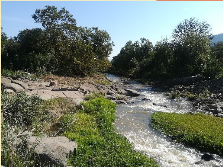
Downstream from Pipe Culvert
