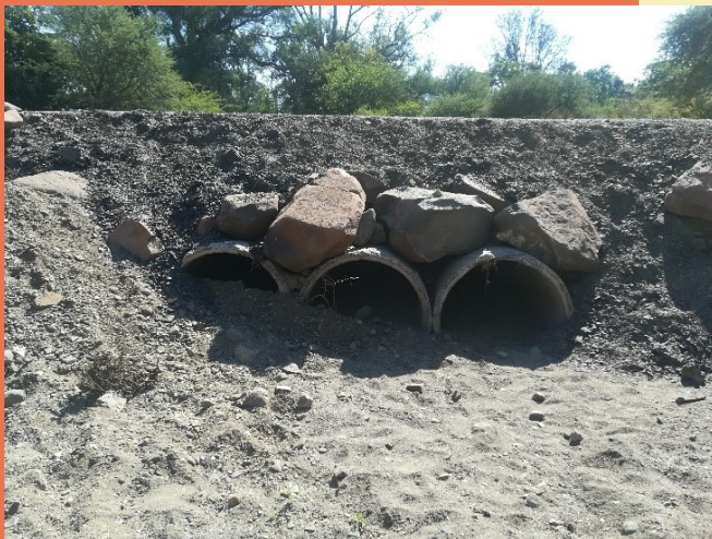
Blocked pipe culverts on the upstream side
